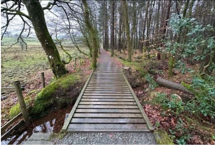
19.01.25 Bridge & Ramp in place
