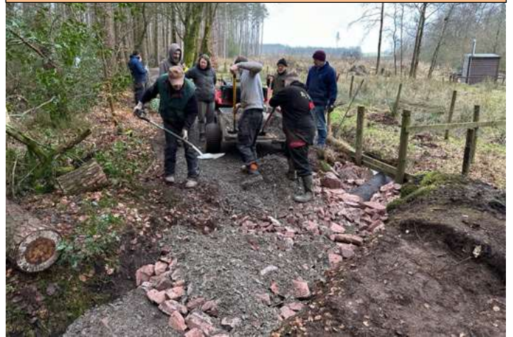
19.01.25 Covering pipe with sandstone and gravel
