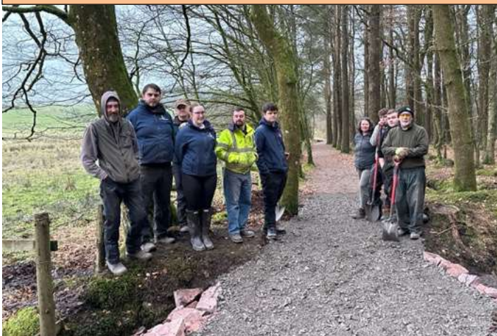
19.01.25 Layer of coarse gravel on top
