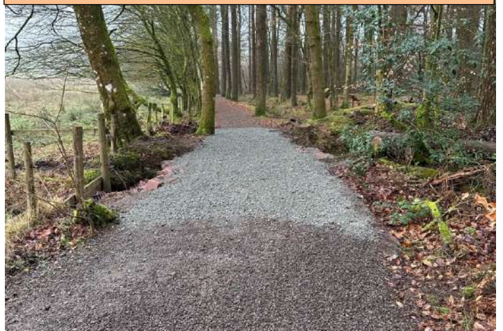
20.01.25 Final surface layer of fine gravel
